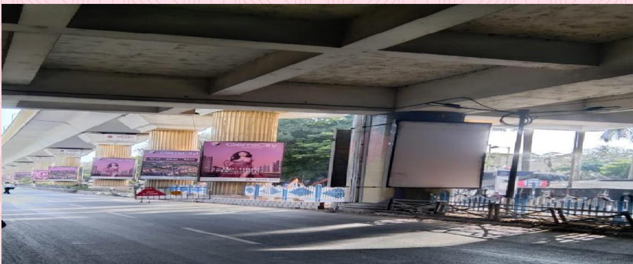
Installing of Iron Fencing in Place of Bamboo (After)
